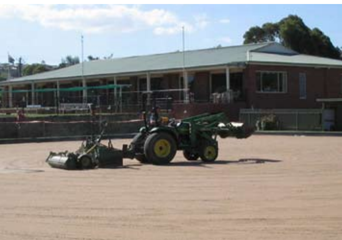
Laser levelling stone layer
