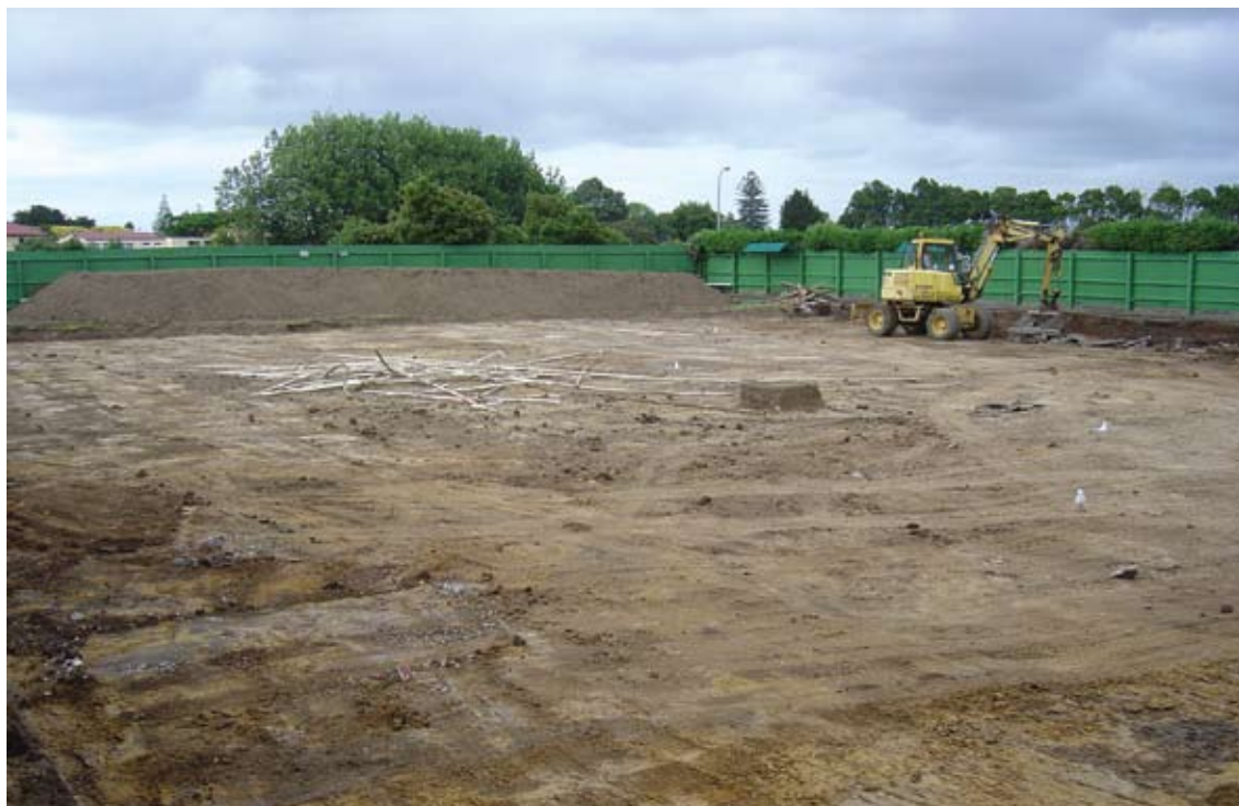
Excavation of an old green prior to laying of sub-base
