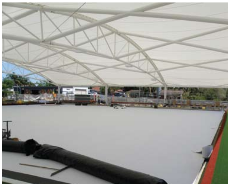
Shock-pad installation prior to synthetic surface
