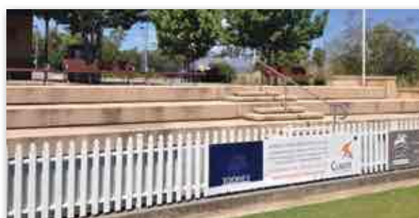
White picket fencing is an aesthetically appealing and traditional cricket ground fencing design
