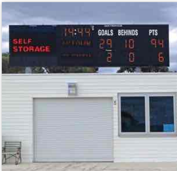
Example of roller door storage with scoreboard mounted to consolidate built infrastructure, Williamstown Cricket Ground (VIC) Image courtesy of insideEDGE Sport and Leisure Planning
