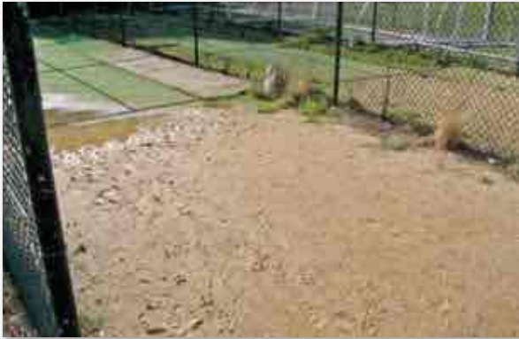
Example of poor quality and unsafe infill materials Image courtesy of insideEDGE Sport and Leisure Planning
