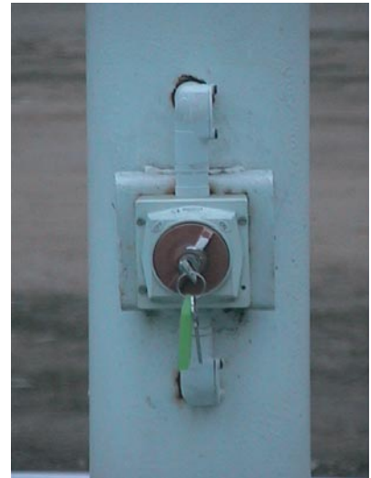
Diagram 1 – The pole is permanently wired from the club switchboard. A key switch at the base of the pole provides lighting control of a playing surface.
