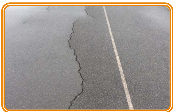
Asphalt cracking
