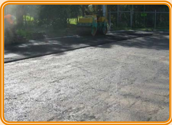
Prime coat on the FCR
