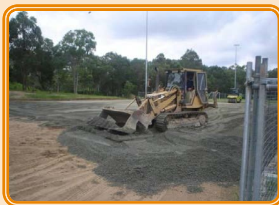
Spreading the crushed rock layer
