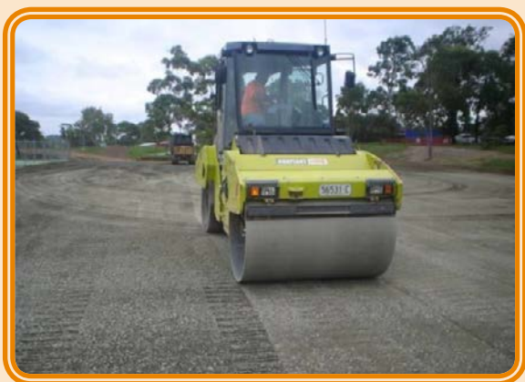
Compacting with a roller
