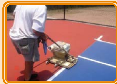
The gravity fed line marking machine method
