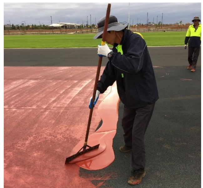
Photo 24: Application of wearing layer over rubber base mat
