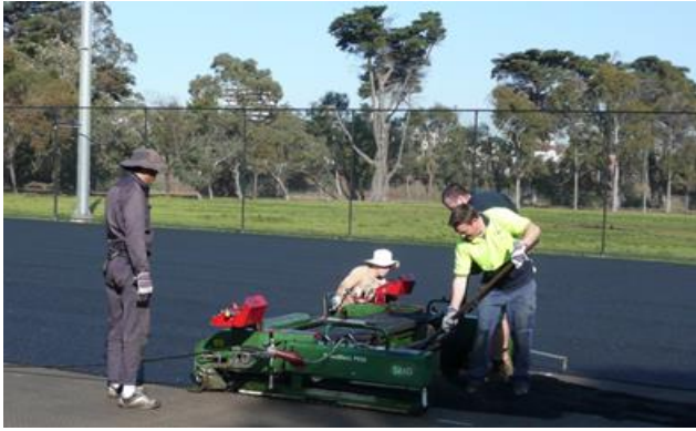
Photo 21: Insitu shockpad being laid (source: Polytan)
