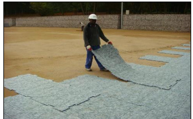
Photo 20: Prefabricated Shockpad being laid (source: Team Sports)
