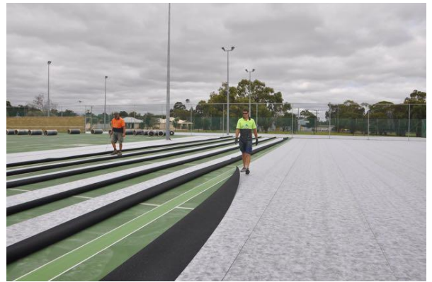
Photo 28: Installation of prefabricated mat system
