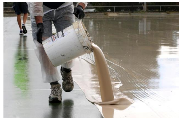
Photo 29: Application of gel system
