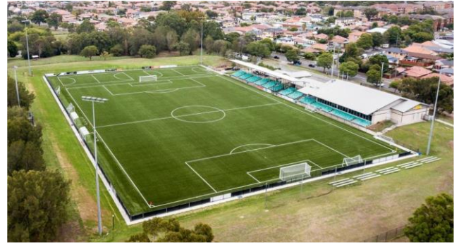
Photo 30: Bicentennial Park (NSW), which was built over a closed tip site with gas capture built into the field
