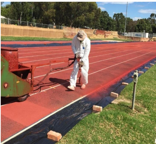
Photo 23: Application of spray coat
