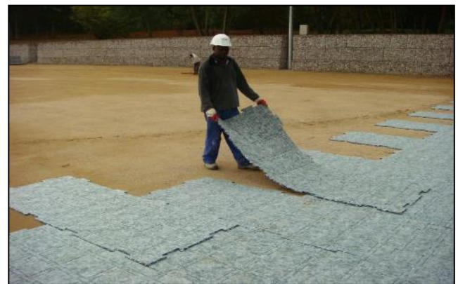
Photo 6: Prefabricated Shockpad being laid (source: Team Sports)
