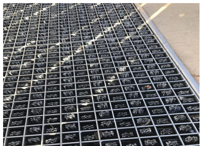
Photo 21: Containment strategy example 2: Pedestrian gate mats that capture the infill
