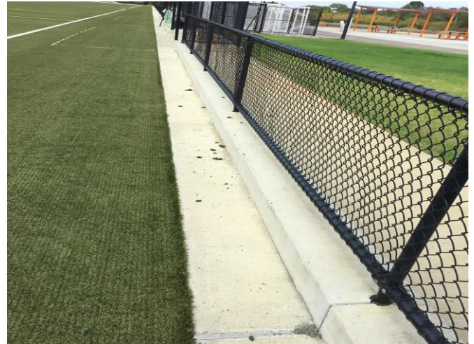
Photo 20: Containment strategy example 1: Curb to reduce the infill being dispersed outside of the field of play
