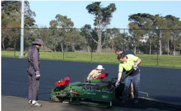
Photo 7: Insitu shockpad being laid (source: Polytan)
