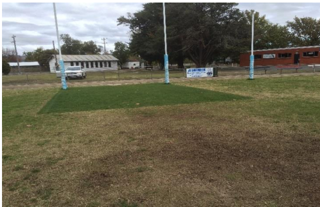
Photo 16: High Wear Area with hybrid surface in goal mouth (source: HG Sports Turf)
