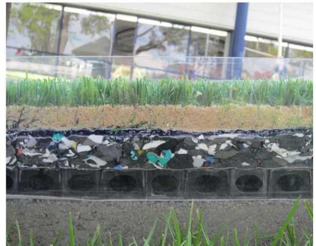
Photo 8: Example of horizontal drainage cell under shockpad (source: Wayne Stuart - City of Swan, WA)
