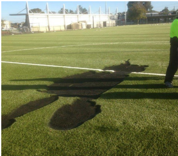
Photo 16: Vandalism can entail a whole section being cut out and replaced
