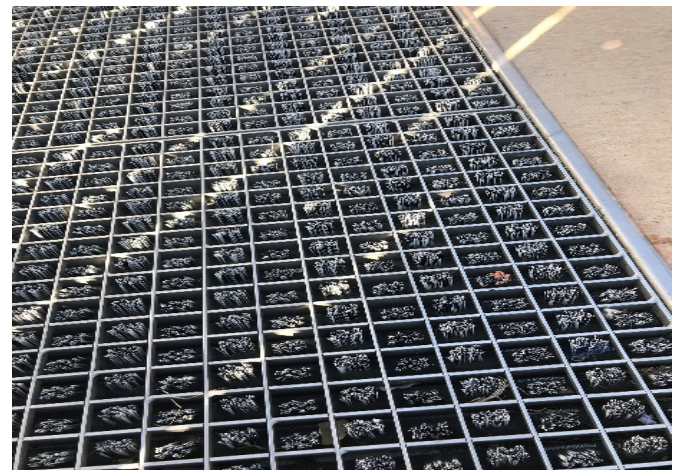
Photo 13: Pedestrian gate mats that capture the infill (e.g. _____)
