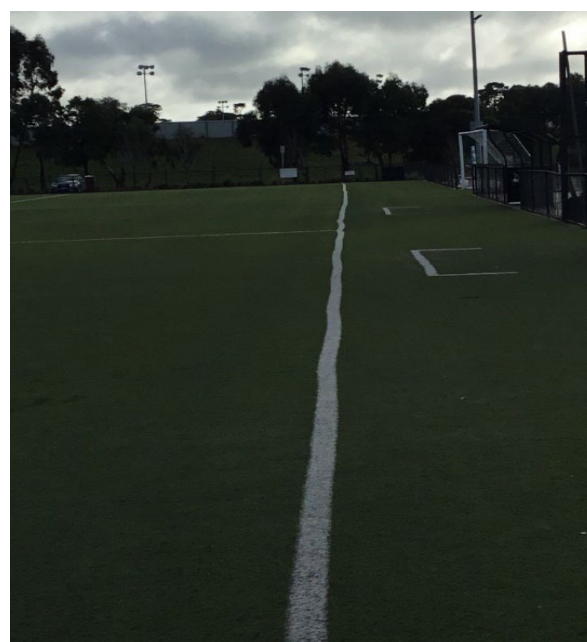
Photo 5: Line movement when there is not adequate infill and the cleaning machine goes over the lines it can stretch the surface
