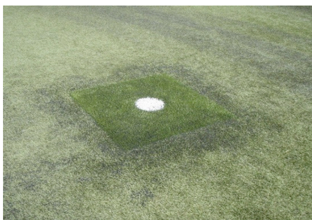
Photo 19: Replacement penalty spot due to excessive wear
