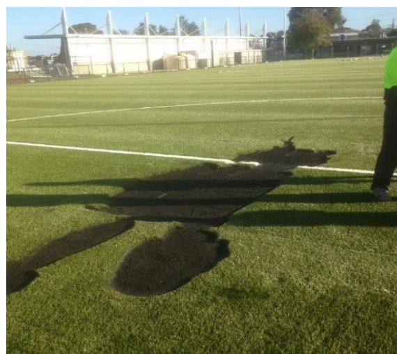
Photo 9.5: Vandalism can entail a whole section being cut out and replaced
