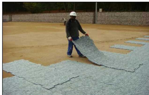
Photo 2.4: Prefabricated Shockpad being laid (source: Team Sports)
