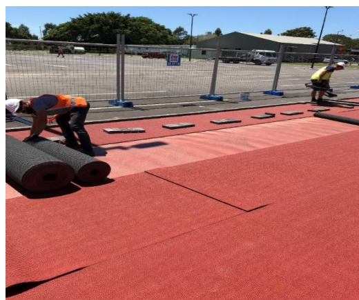
Photo 2.9: Rolling-out prefabricated synthetic surface
