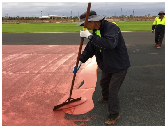
Photo 2.8: Application of wearing layer over rubber base mat
