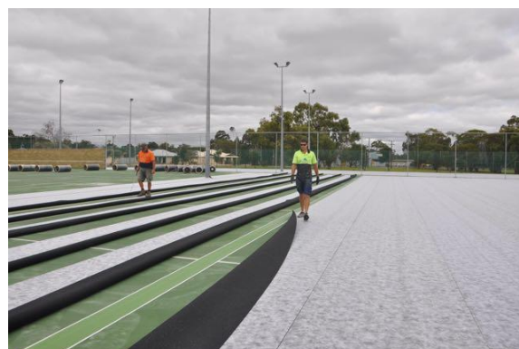
Photo 2.12: Installation of prefabricated mat system
