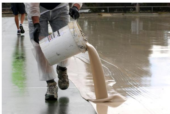
Photo 2.13: Application of gel system
