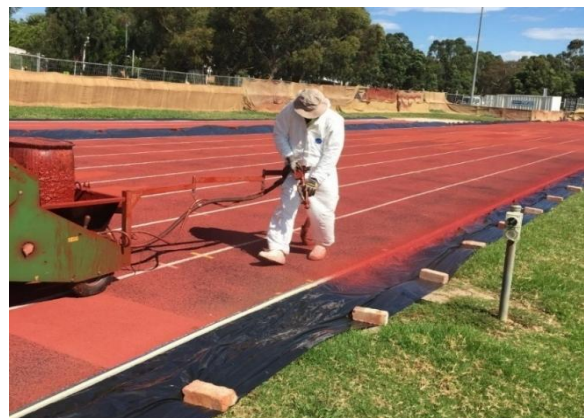
Photo 2.7: Application of spray coat
