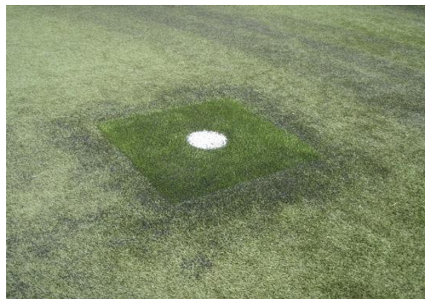
Photo 9.8: Replacement penalty spot due to excessive wear
