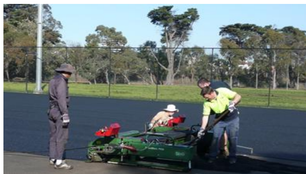
Photo 2.5: Insitu shockpad being laid (source: Polytan)
