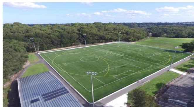
Photo 3.4: Lane Cove Council installed Blackman park with synthetic turf and Brock infill (woodchip) and the temperature is significantly cooler
